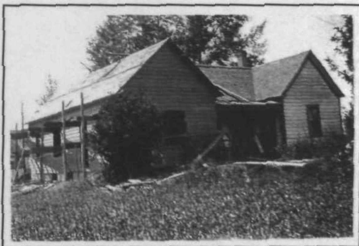
NEW PART BEING BUILT ON
